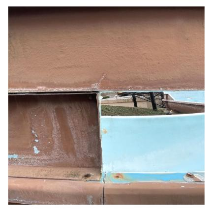
Corrosion on fasteners and missing fasteners were noted in several locations, including areas where the splash guard failed.
