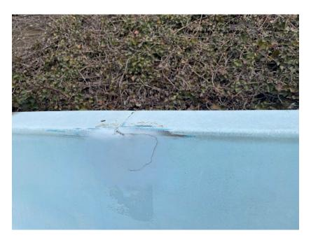
• Downstream end of damaged splash guard. Note crack in panel above on close -up.
